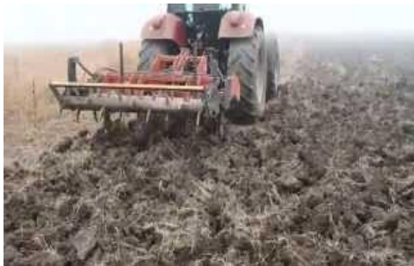
Fig.2. Execution of scarifying and rolling work. Source: authors.
