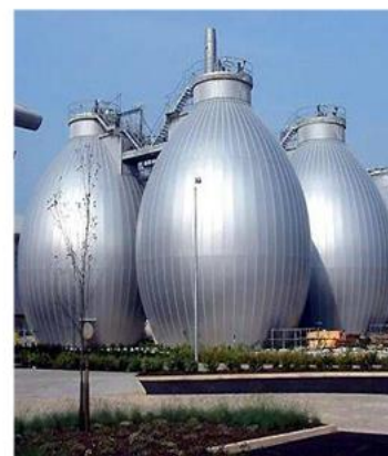
Fig. 5. Diagram of sludge processing in mechanical-biological treatment plant [19] and egg-shaped sludge digesters [23]
