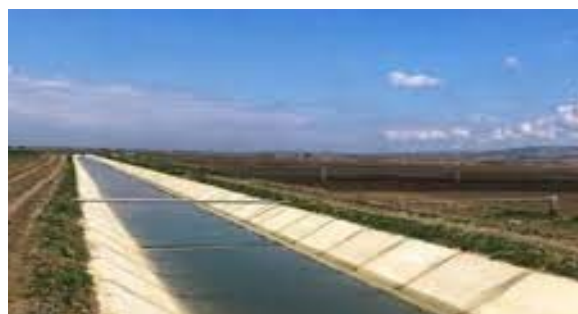
Figure 2. Rehabilitated irrigation channel
