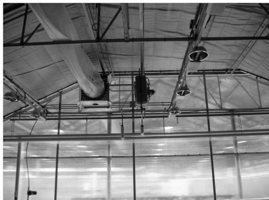
**Fig.8. – Unit heaters, (Ponce et al., 2015)**
